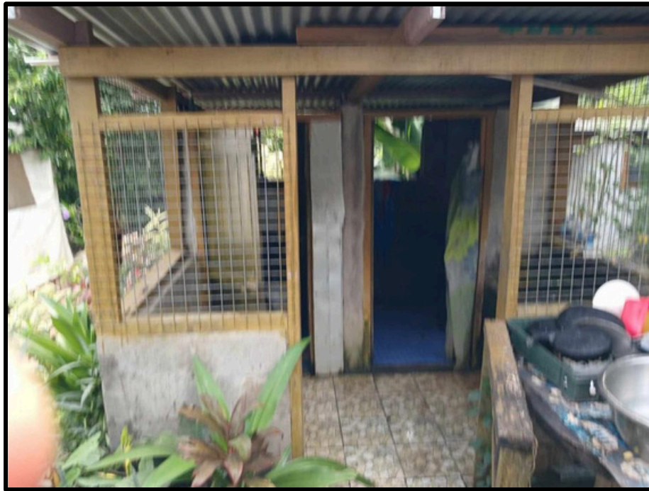
Figure 8. Bathroom & Toilet Block (Naiwasetawa, 2024)
